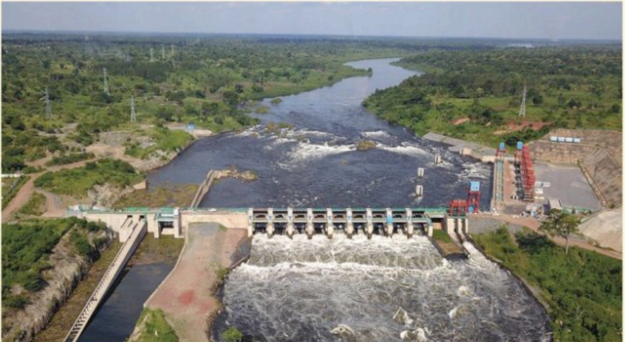
Karuma Power Generation Dam
