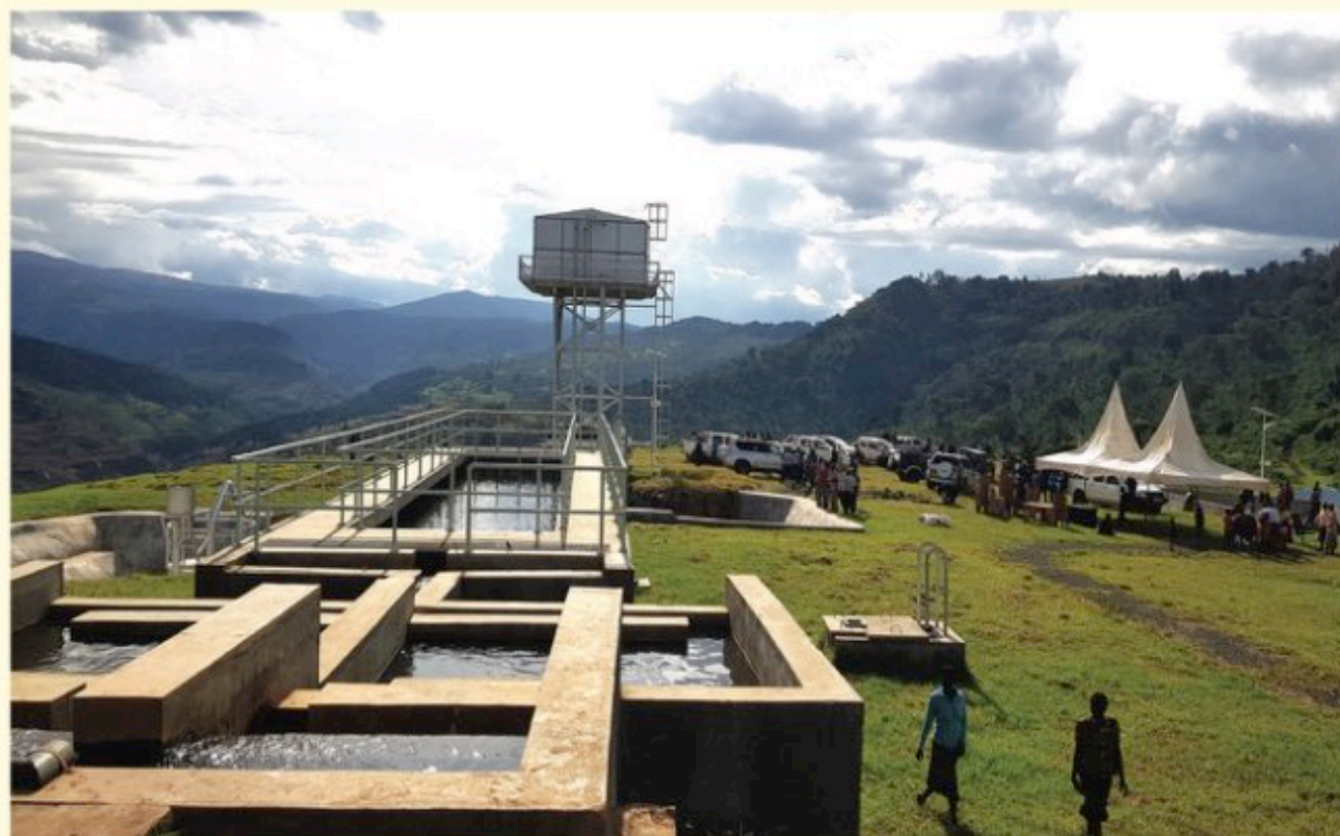
Bukwo Water Treatment Plant
