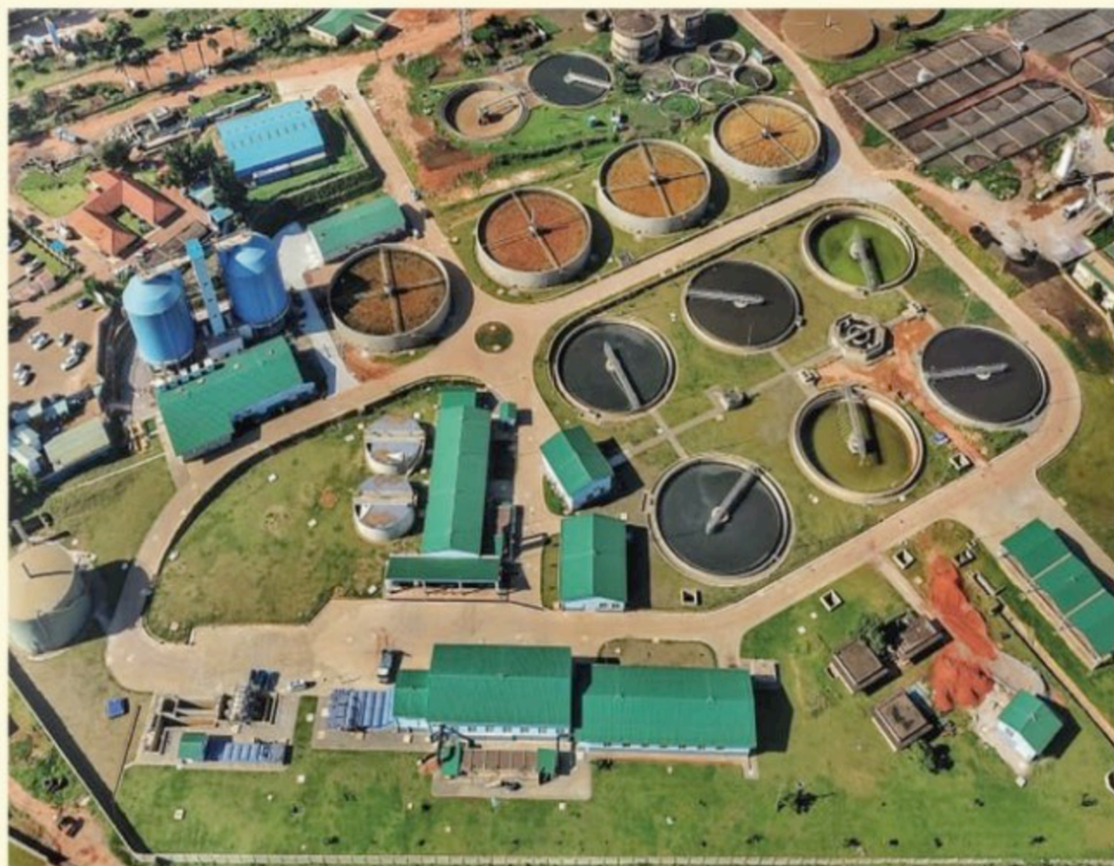
Construction works at Katosi water treatment plant
