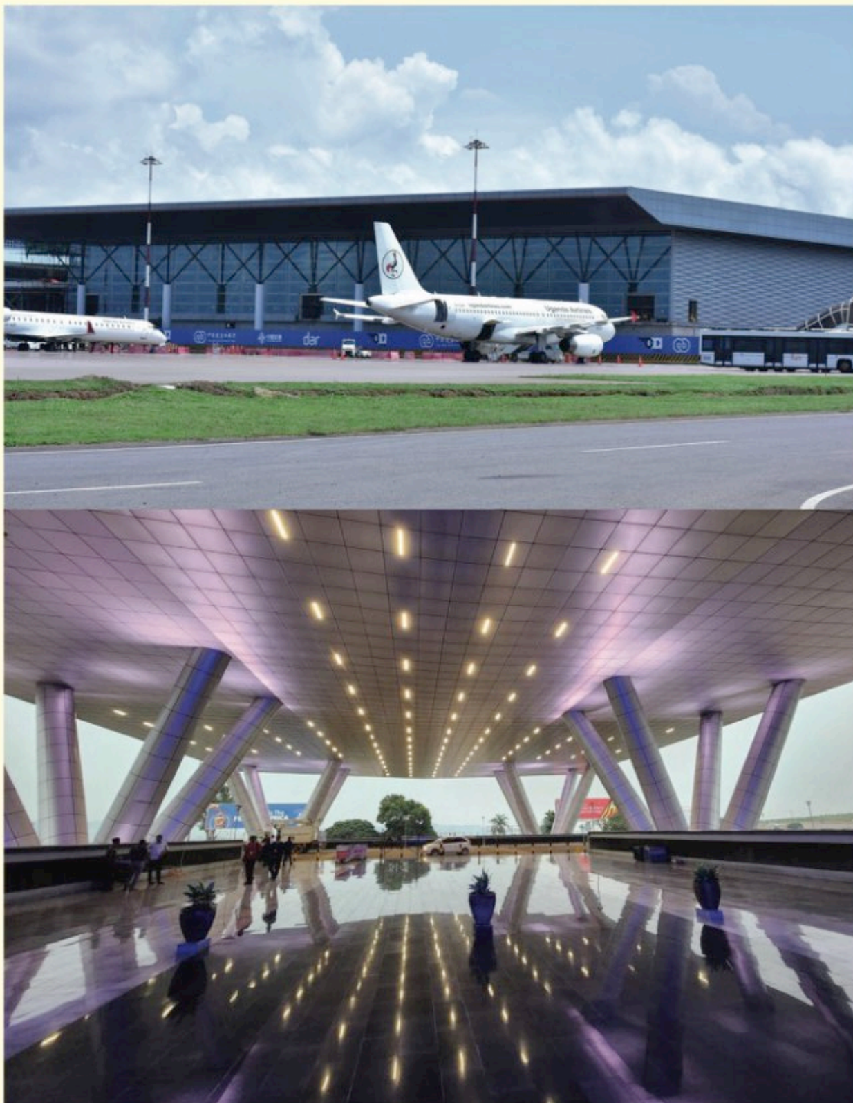
The newly rehabilitated Entebbe International Airport
