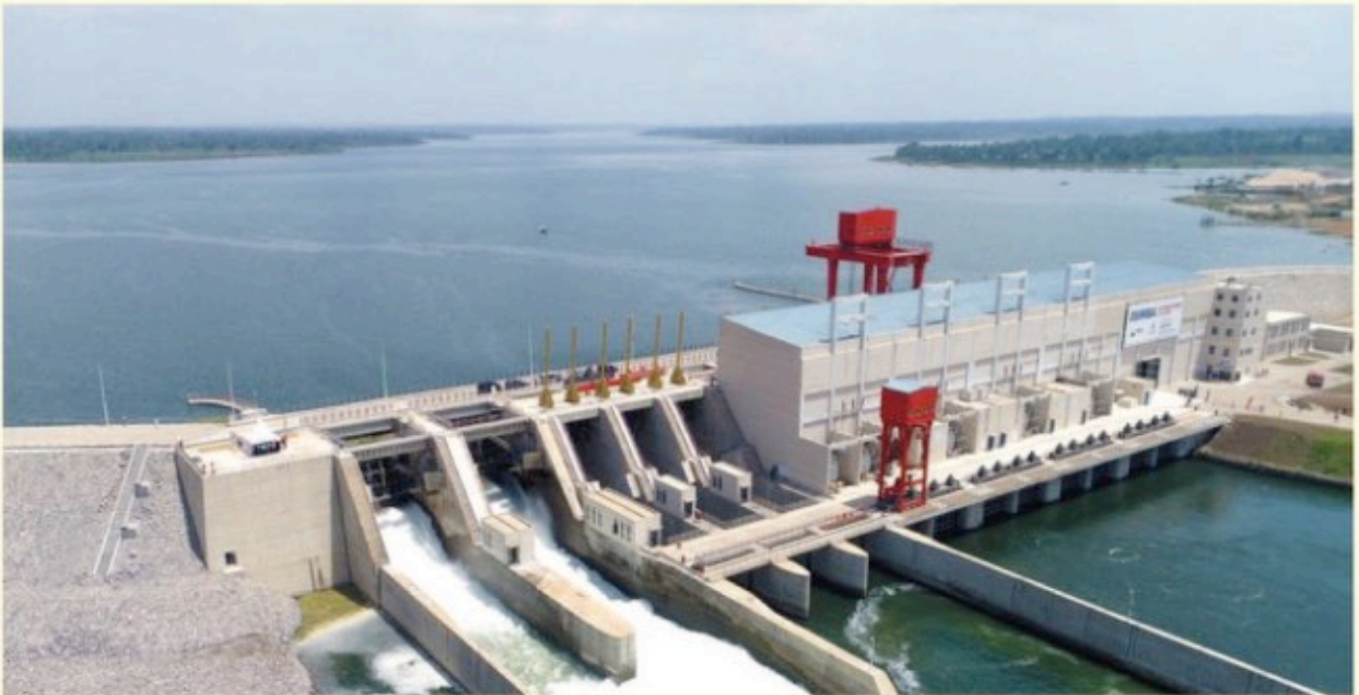
Isimba Power Generation Dam
