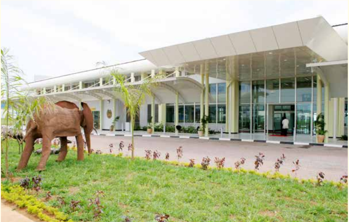
The new wing of the Entebbe Airport
