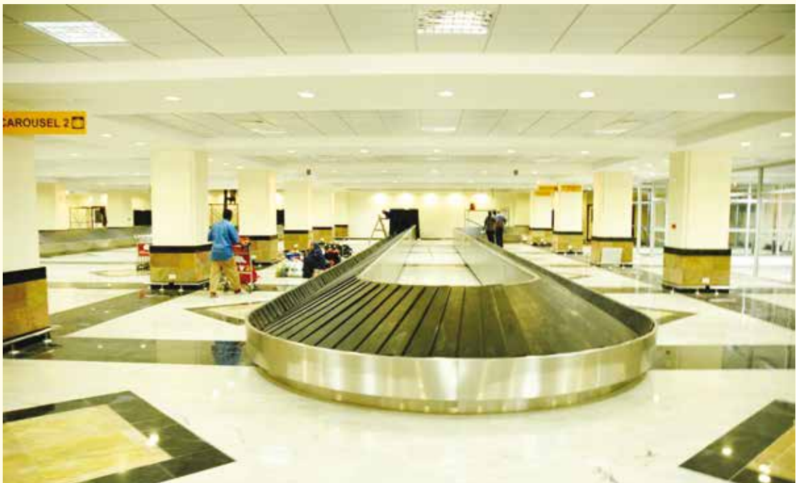
The new Baggage Conveyor at Entebbe Airport
